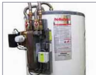
SHWM mounts easily to tank or nearby wall
